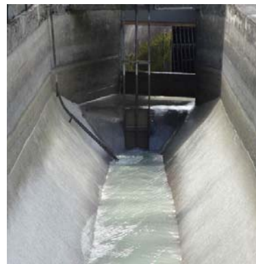
Figure 3 - Sand trap during the drawdown flushing of the left basin, seen in flow direction.
