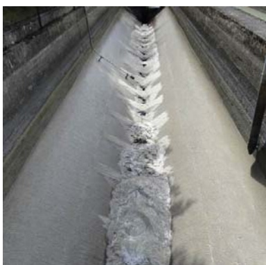
Figure 4 - Deposited material remaining above the sediment excluder at the end of drawdown flushing (left), and wooden planks after the final cleaning (right).
