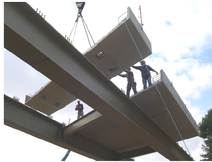
Fig. 1.3: Positioning of prefabricated segments over steel girders [Artéfac 2008]
