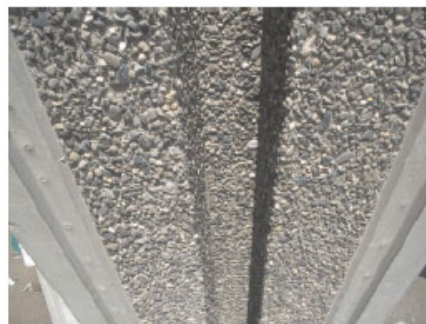
Fig. 1.8: Inner rib of slab with roughened surface [Dauner 2006]
