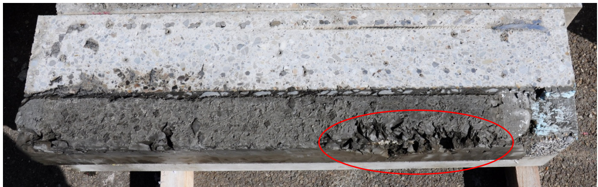
Fig. 3.58: Block of specimen PR100_3, missing part of cement grout
