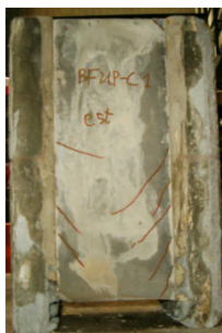
Fig. 3.12: UHPFRC-cement grout specimen, with excessive initial cracking.
