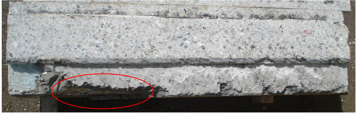
Fig. 3.57: Cracking of concrete block of specimen PR100_3 close to the interface
