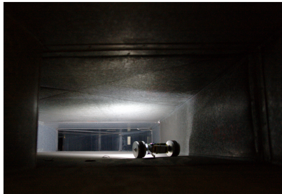
Figure 3.19: Cy-mag 3D II lighting the air duct.
