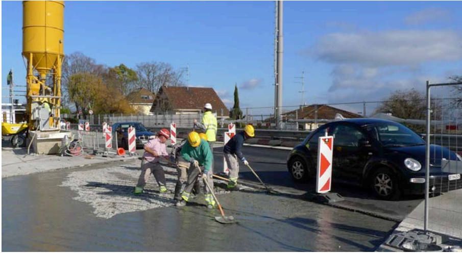
Figure 6: Underpass “Creux de Genthod” – nearby Geneva (CH), 2010, rehabilitation of a bridge deck with SH-UHPFRC, slope 5 %, average external temperature 5 °C
