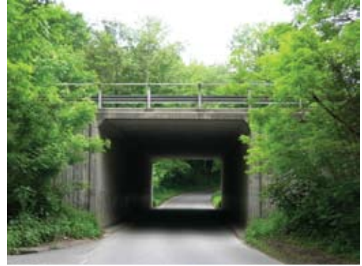
Figure 5. A: Underpass of a highway.
