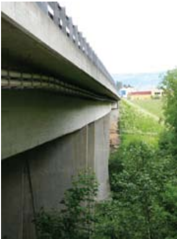
Figure 7. C: Highway viaduct.
