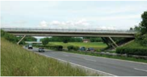
Figure 6. B: Overpass of a highway.
