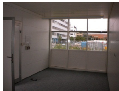
Fig.2 Interior view of the standard double glazing module at the EPFL campus (Switzerland).
