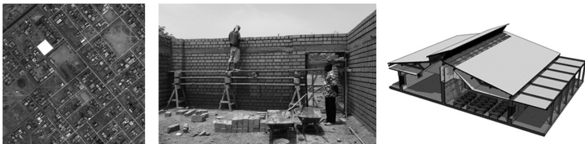
Figure 5: FITIMA centre: the aerial view of the neighbourhood, the construction site on February 2011 and the proposed optimized roof model for the educational block
