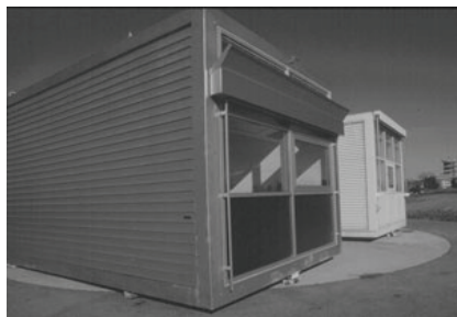
Fig.1 Outside view of the two test modules on the EPFL campus. The test module on the left side contains integrated anidolic systems (IAS) and the test module on the right side is equipped with a standard glazing window.
