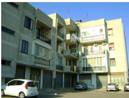
Figure 1. View of the case study building
