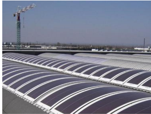
Fig. 2: Examples of thin film silicon module integration; (left) Demonstrator realized at the PVLab of EPFL, (right) Flexible modules produced and commercialized by Flexcell on the roof of an industrial building.
