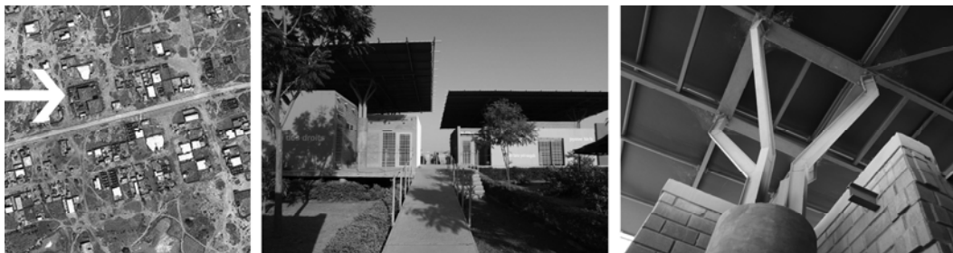
Figure 2: The case study - CBF centre for the well-being of women, a European Commission financed and NGO supported educational building located in the northern suburb of Ouagadougou, aerial photo of the project, the exterior view and its roofing system
