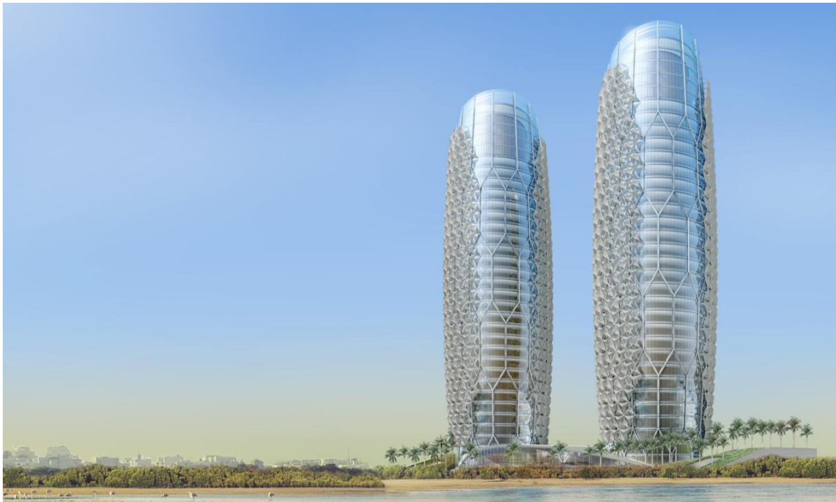
Figure 01. Al-Bahr ICHQ Towers; Emerging from the landscape, the energy and structural performance driven design dictated the organic form and geometric formation of the surrounding kinetic shading components.
