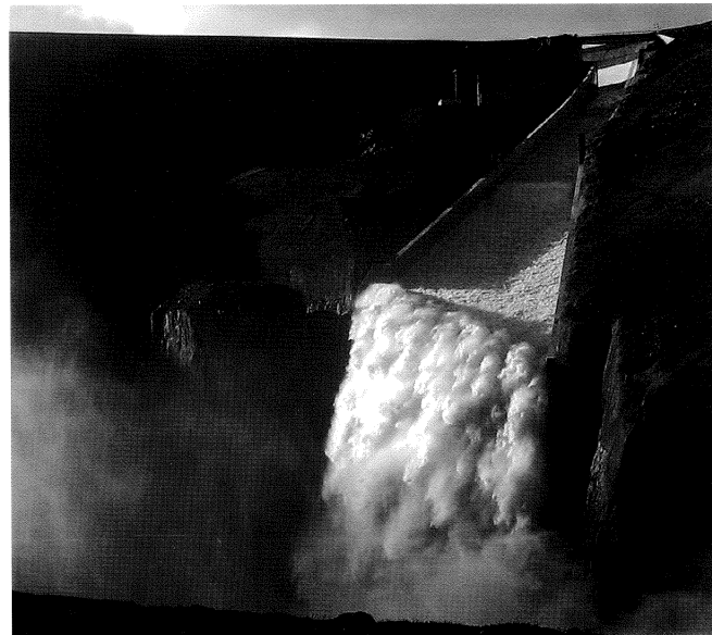
Figure 10. Prototype spillway flow and jet pattern for approximately 200 m 3 /s (courtesy Landsvirkjun).
