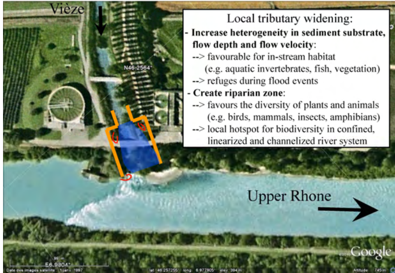
Figure 6-2: Confluence of the channelized Upper Rhone and Vièze Rivers. Local widening is schematic illustrated and its main objectives are listed.
