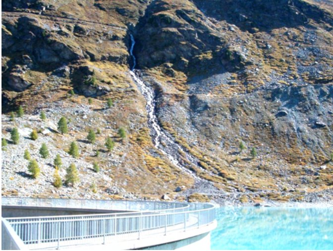
Figure 3.16 Water transfer from a neighbor catchment with a head of 170 m (Tourtemagne)
