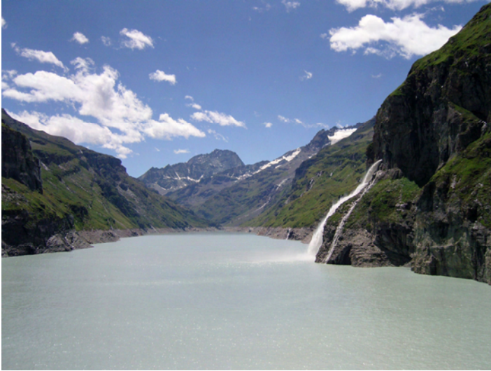
Figure 6.1 Reservoir of Mauvoisin with the water transfer tunnel from Corbassière and Séry (Source: Wikipedia.org, author: Goudzovski)
