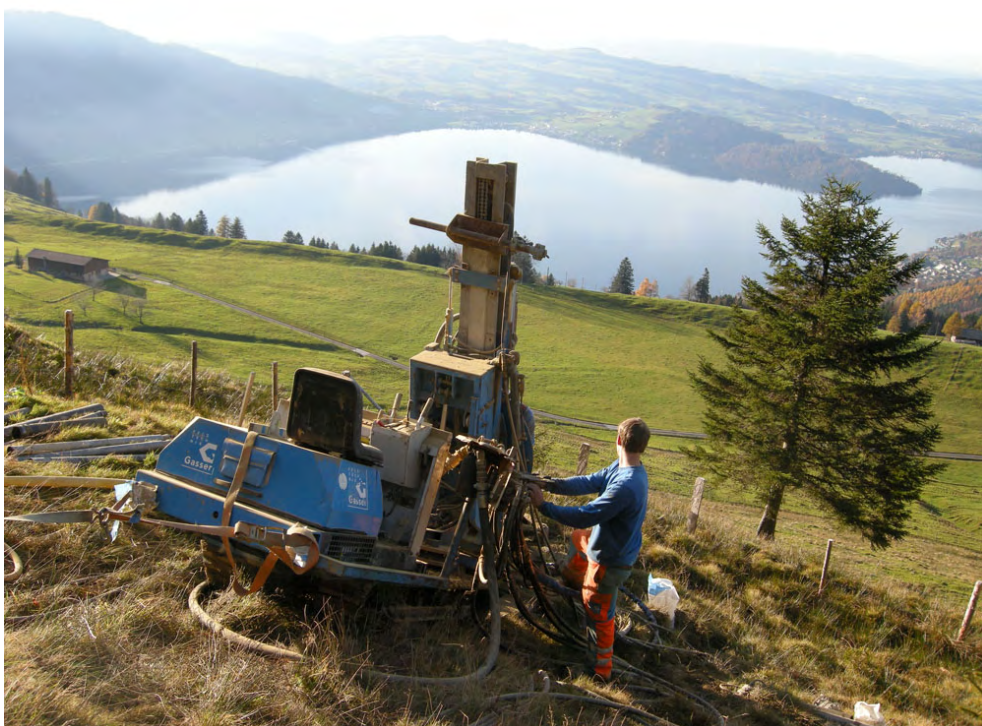
Figure 4.7: Photograph of the drilling rig used on the Rufiberg slope, November 2010.
