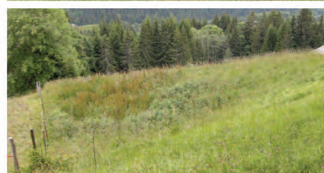
Swampy areas above the Pont Bourquin landslide, 9 July 2009
