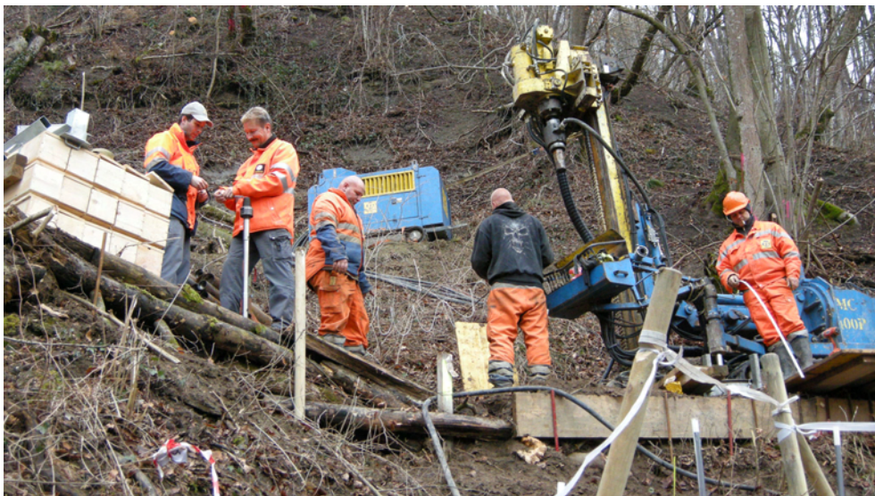
Figure 4.5: Photograph of the drilling platform and drilling rig located above the test site, March 2009.
