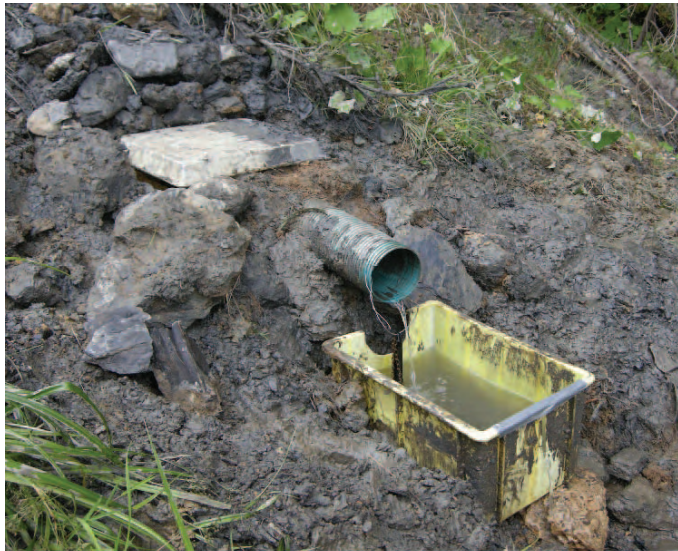
Weir of spring 32, middle part of Pont Bourquin landslide, 28 June 2010
