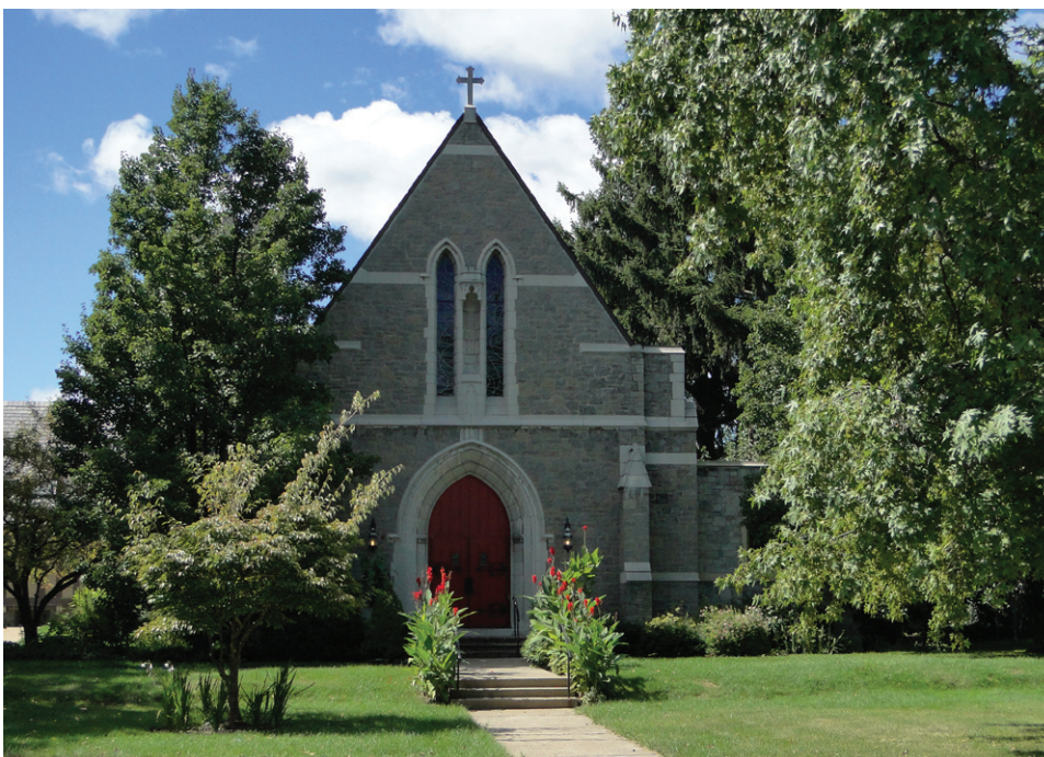
fig. ROC 11. St. Thomas Episcopal Church. Winton Road et Highland Avenue.
