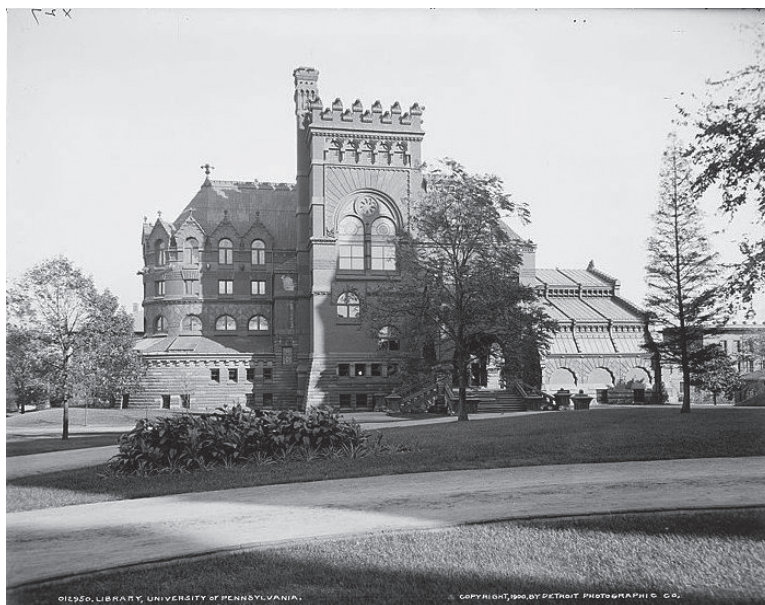
fig. II. 13. Frank Furness, Fisher Fine Arts Library, l'Université de Pennsylvanie, Philadelphie, 1890. La photo : Auteur inconnu, Library, University of Pennsylvania, Philadelphia, Pennsylvania, from the west, 1900. Source: Library of Congress, Detroit Publishing Company Photograph Collection, http://memory.loc.gov/service/pnp/det/4a00000/4a08000/4a08400/4a08444v.jpg
