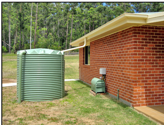
Figure 1: Plastic rainwater tank
