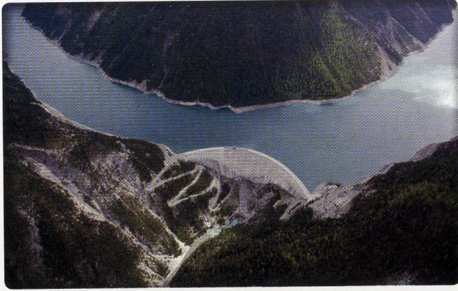
Punt dal Gall, a 130 meter-high arch dam in Switzerland and its associated 393 MW hydro facility, feature in the pre-conference and post-meeting tours.
