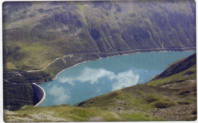
Nalps Dam is undergoing intensified monitoring as a result of construction of the Gotthard Base Tunnel. This railway tunnel beneath the Alps was completed in 2010.
