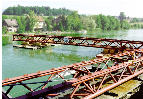
(b) Aarwangen bridge (canton of Bern, Switzerland) composed of two planar tubular trusses with K-joints (2 × 48 m spans)
