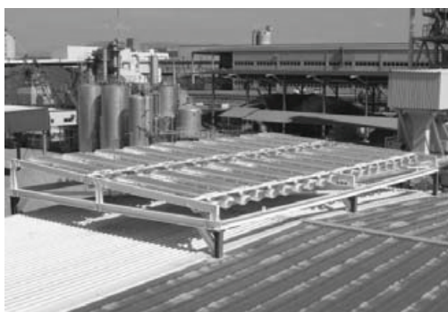
Fig. 5. The solar field made of 20 SRB solar thermal collectors installed at COLAS premises.
