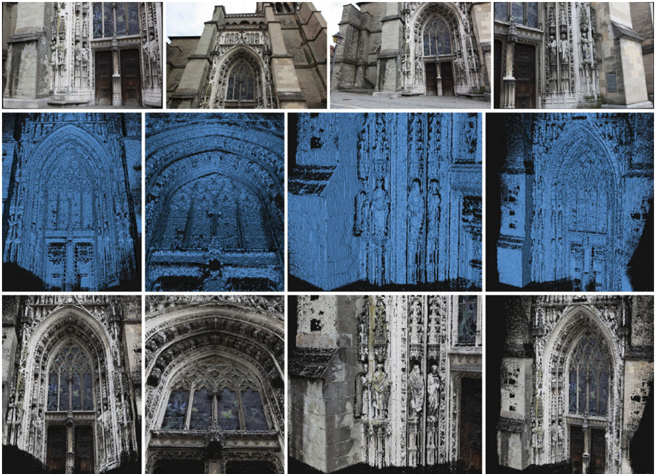
Fig. 7 Cathedral portal reconstruction. The 3D point cloud was constructed in 9.2 min from 13 21-Megapixel images and contains 20.3 million points. Top row Some example images of the data set. Middle row
