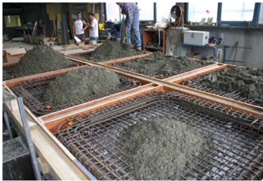
a) Concrete casting
