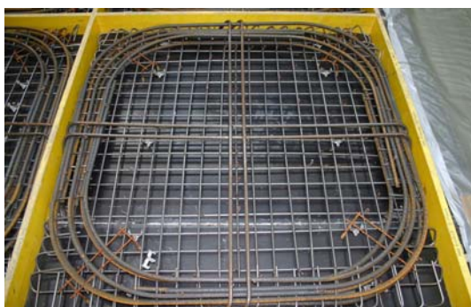
c) Dowel steel reinforcing bars
