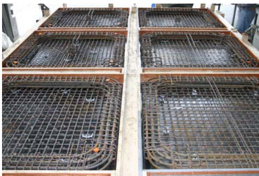
b) Formwork and reinforcement
