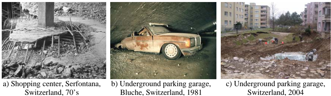
Figure 1.1: Structural collapses due to the punching shear failure
