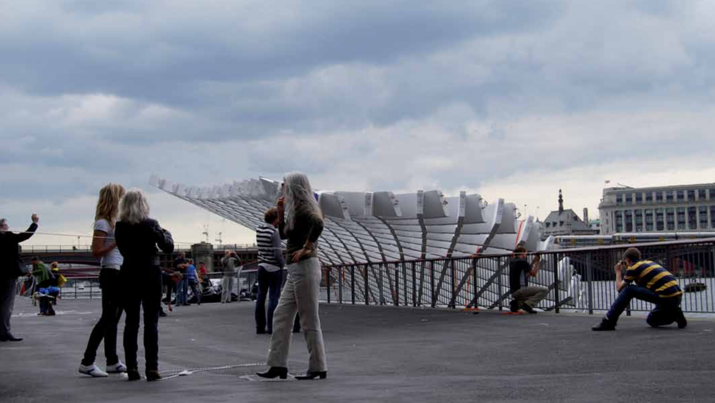
Overflow at high tide
