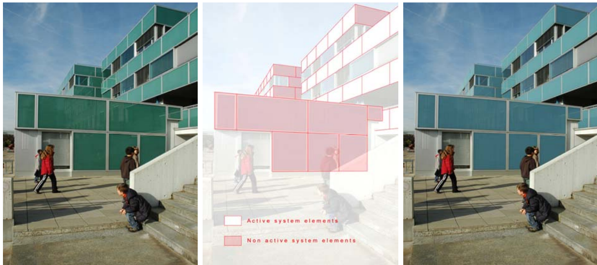
Fig 7.a (left): Primary School in Pully, CH: building renovation (Devanthery & Lamunière 1998-99) using coloured glass cladding over opaque envelope parts; Fig. 7.b (center): The standard glazing could be replaced by the new glazing. In the exposed facade areas they would be used as collector glazing and in the non exposed ones they would be used as facade cladding over insulation. Fig.7.c (right): Integration simulation, using a blue coated acid etched glazing with small squares pattern. The building still looks very similar to the original: the facades are homogeneous, and the solar system doesn't affect the building appearance.
