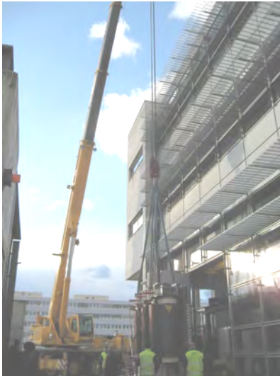
Fig. 4.3.1 Unloading of one of the transformer (19 tons).
