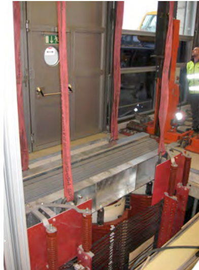
Fig. 4.3.2 Unloading through the trap door into the basement.
