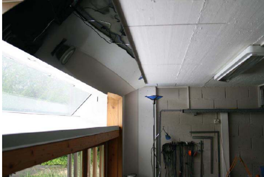
Figure 8.9: The anidolic system that redirects daylight to the interior of the rooms.
