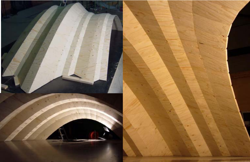
Figure 3: Shell structures made out of timber block panels
