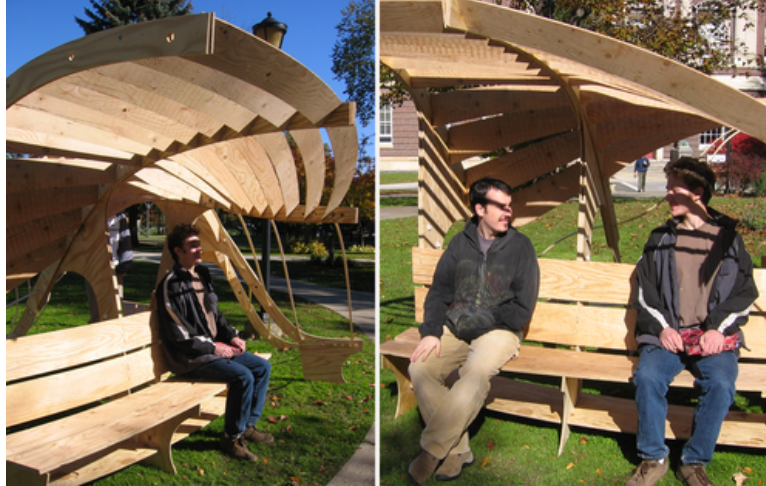
Fig. 2. Sunlight penetrates the louvres of this architectural studio project in an unanticipated way, causing discomfort. An interactive daylight renderer could have predicted this problem, allowing the designer to optimize the orientation of the louvres.
