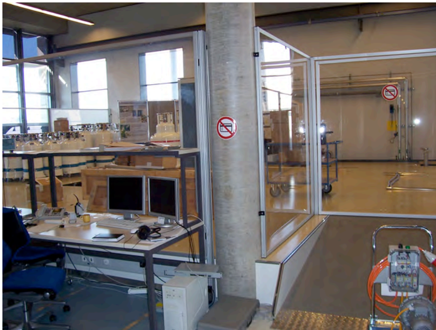
Fig. 3.7.5 View of the entry ramp to the test facility security enclosure as of 21 September 2005. Inside the clear barrier are stored, temporarily, the liquid Helium dewars (blue striped – 66l, 100l, red striped – 250l) and 2MW transmission line components (in boxes).
