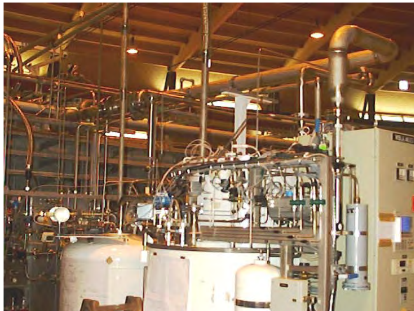
Fig. 3.6.6 Installation of the HELIAL-100 coldbox and the 500 liter Dewar
