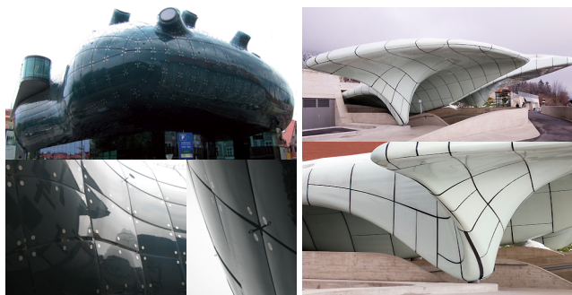
Figure 2: Projects involving double-curved panels where a separate mold has been built for each panel. These examples illustrate the importance of the curve network and the challenges in producing architectural freeform structures. (Left: Peter Cook and Colin Fournier, Kunsthau, Graz. Right: Zaha Hadid Architects, Hungerburgbahn, Innsbruck.)
