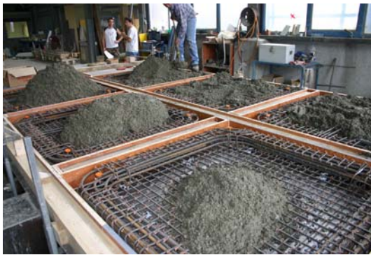
a) Concrete casting
