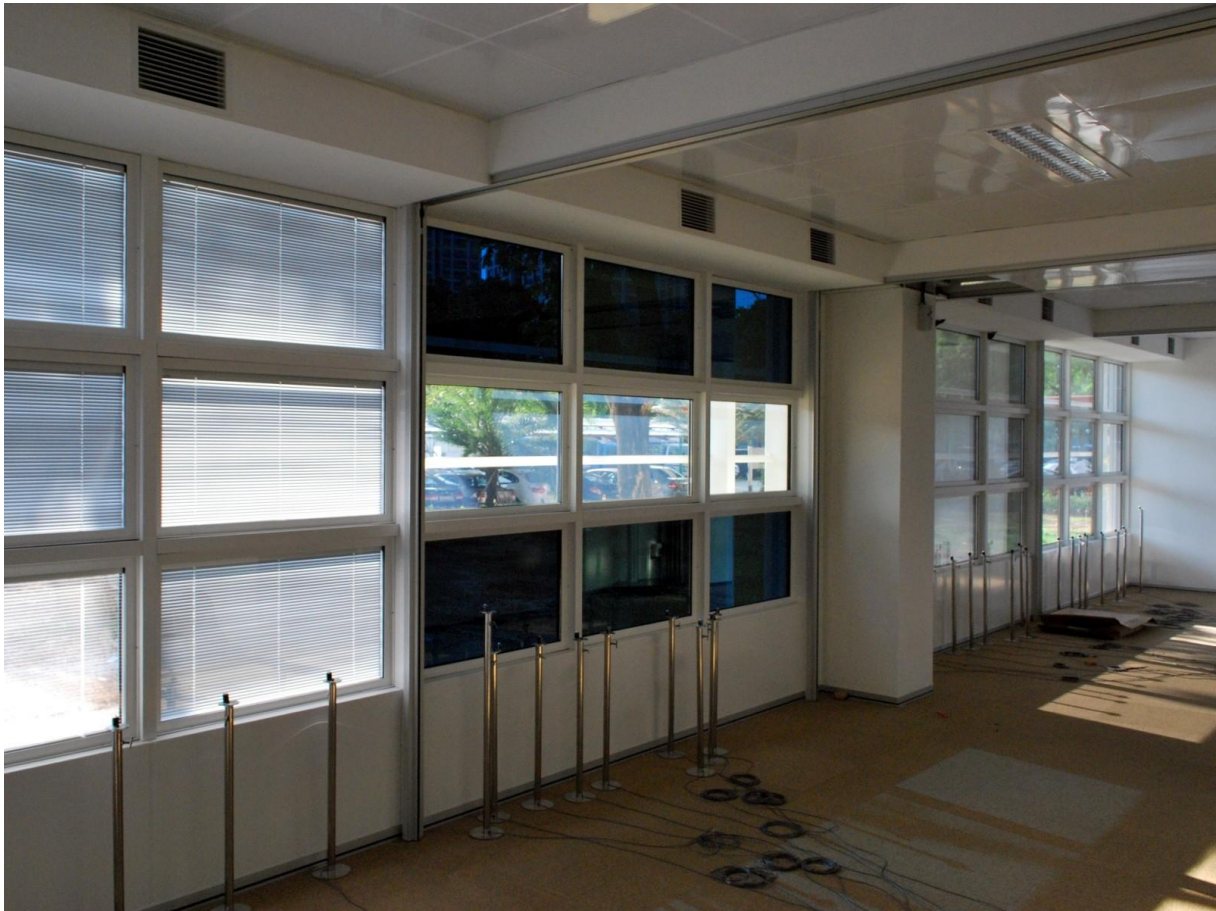
Figure 1: Facade as seen from inside with partition walls opened. From left to right: glazing integrated blinds, electrochromatic glazing, aSi photovoltaic glazing, and clear glass.
