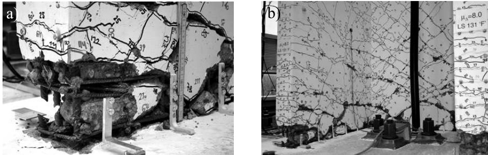
Figure 3.12. TUA: West flange end showing the ruptured D12 bars (a) and the lower part of the West flange and the web (b) at Position F during the diagonal cycle with \mu_{\Delta} = 8.0 (point of failure).
