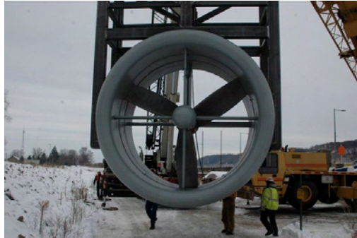
Figure 1: Typical hydrokinetic turbine (source: Alternative Energy Info, www. www.alt-energy.info)
