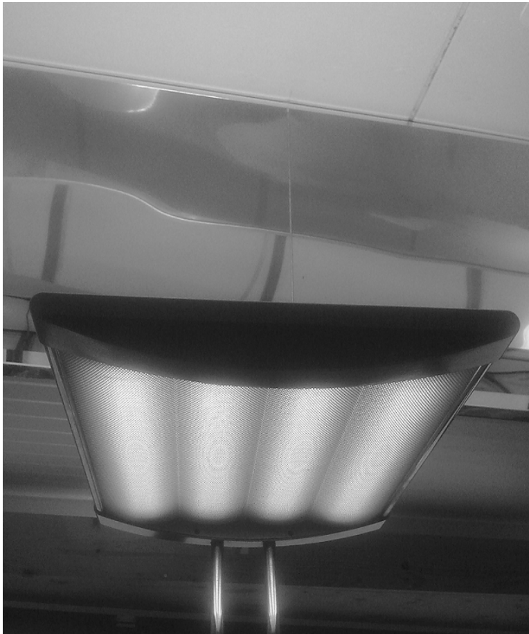
Figure 3.12: Indirectly emitting luminaire. - The figure shows a free-standing luminaire for semi-indirect lighting.
