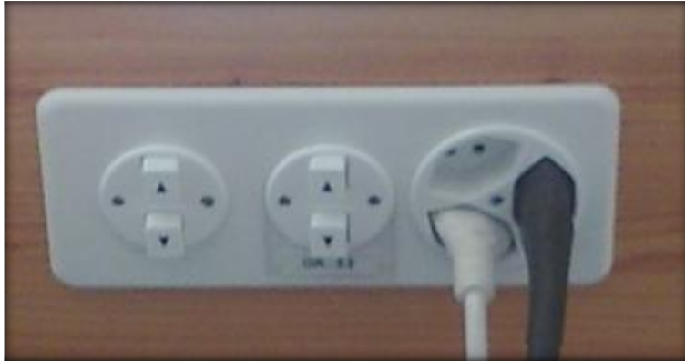
Figure 2.17: Switches for controlling the LESO building's external blinds. - This photograph shows the four blind switches installed in every room of the LESO building.
