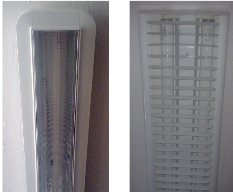
Figure 3.11: Directly emitting luminaires. - The figure shows one luminaire for direct lighting shielded by an acrylic glazing (left) from the 1990's and one shielded by several vertically oriented battens (right) from the 1980's.
