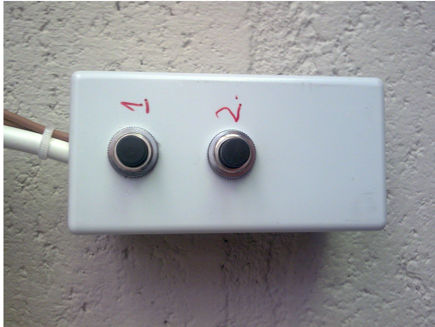
Figure 5.8: Touch Dim push button couplers. - The figure shows the two push button couplers associated with the Touch Dim lighting control.
