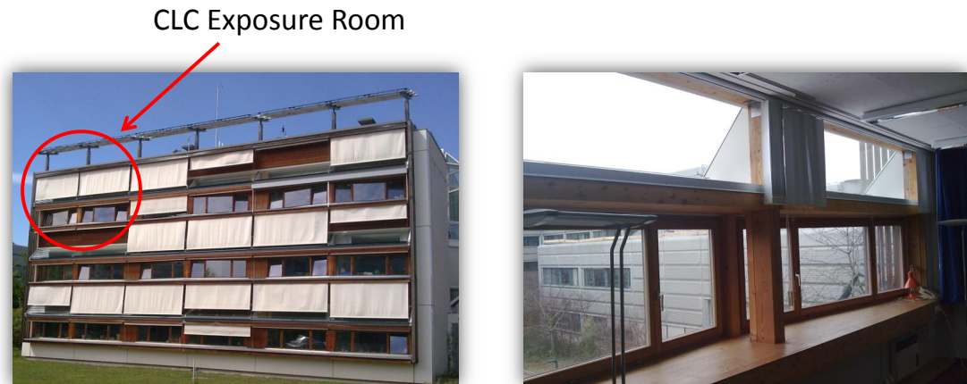
Figure 9.1: Controlled Lighting Conditions Exposure Room - The photograph on the left shows the location of the CLC Exposure room on the second floor of the LESO building in Lausanne. An inside view of the room's two ADS is shown in the photograph on the right.
