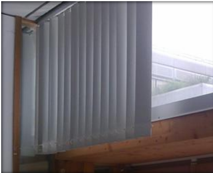
Figure 2.15: Internal Californian blinds for glare protection. - The figure shows the internal Californian blinds for manual glare protection installed in the ADS-equipped office rooms of the LESO building.
