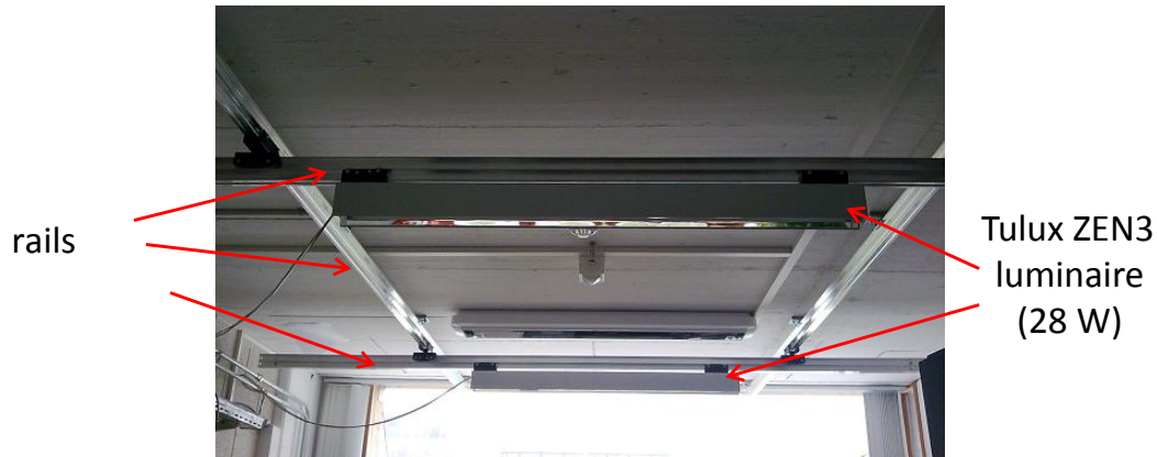
Figure 5.1: Ceiling-mounted rail system. - The figure shows the rail system with two mounted Tulux ZEN3 luminaires.
