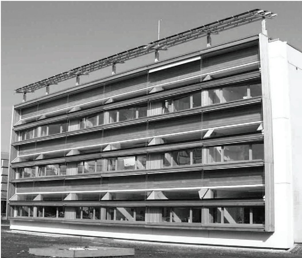
Figure 2.1: The Anidolic Daylighting System - This photograph shows a southern view of the LESO building with the façade-integrated Anidolic Daylighting Systems (ADS).
