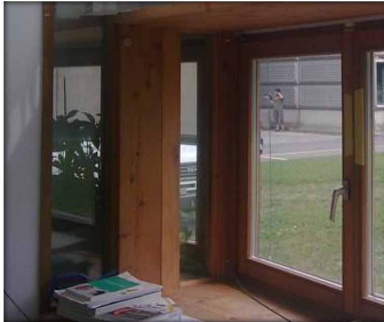
Figure 2.16: Small lateral opening between two LESO office rooms. - The figure shows the small lateral openings between two office rooms which can sometimes lead to temporary discomfort glare.
