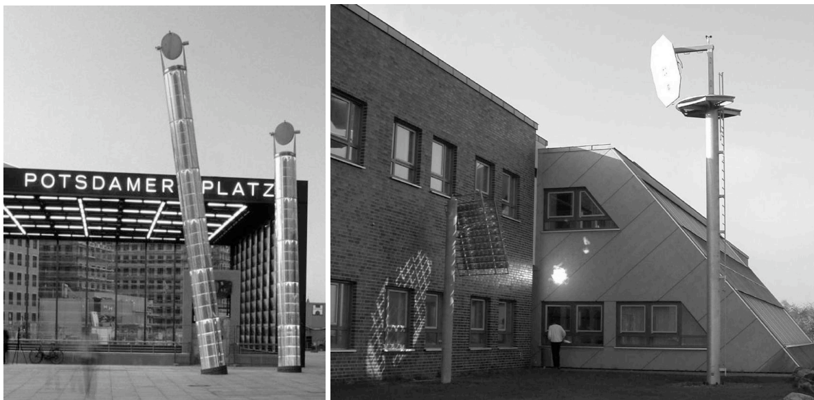
Figure 2: Heliostat-lightpipe systems (left: heliobus® system at Potsdamer Platz, Berlin, right: Daylighting system with EGIS heliostat at Solar-Institut Jülich /2/).
