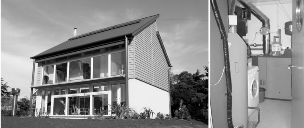
Figure 1 BASF House, South Façade, sunspace(left) and plant room (right).
