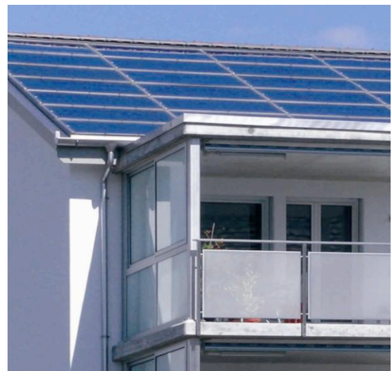
Figure 1: A renovated apartment building in Staufen, CH with roof-integrated PV, new deeper balconies and uninterrupted insulation (www.setz-haus.ch Photo AEU)
