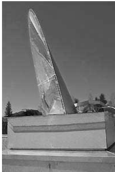
Figure 1: The heliobus® mirror installed at the school building Boppartshof in St. Gallen, Switzerland (Source: www.heliobus.com ).
