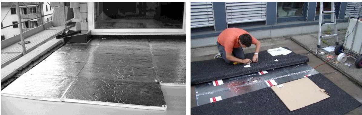
Figure 2: Example of a slim balcony insulation with VIP giving equal levels for indoor and outdoor zones (Left, photo from 2003. Today, panels for on-site installation are often shipped with glued-on protection layers.) Installation at the test site (right).
