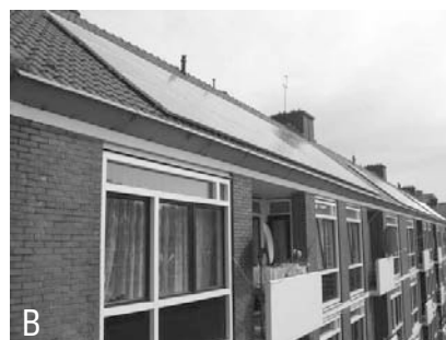
Figure 2: examples of installation of solar thermal collectors and photovoltaic modules
