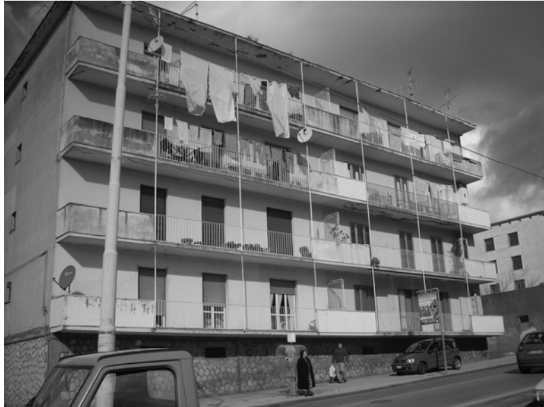
Figure 4 - A picture of the building chosen for the rehabilitation
