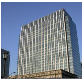
Figure 1: Western façade of the building.
