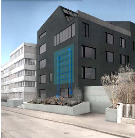
Figure 5: B35 building rendering with a sketch of the active insulation piping system shown over one wall
