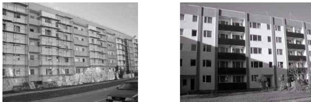
Figure 3: During and after insulation of the building.
