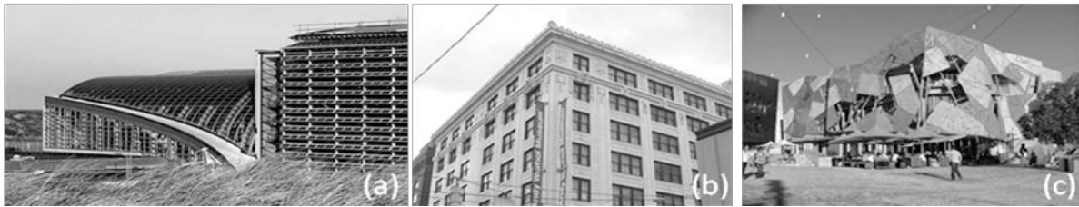
Figure 4: reference buildings, 4a the ECN building in Petten, the Netherlands; 4b the Andy Warhol Museum in Pittsburgh, USA; 4c Federation Square building in Melbourne, Australia.
