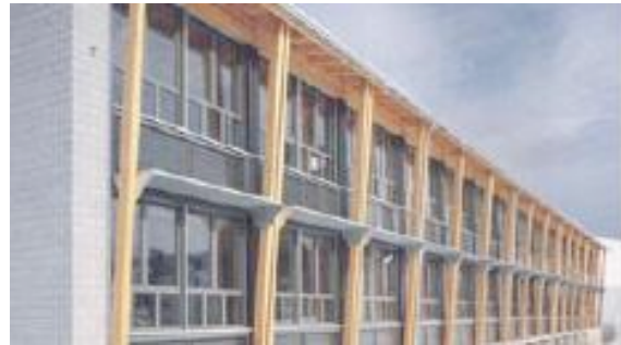
Figure 2: integration of solar thermal collectors into the balcony of the Upper Stage Centre (D).
