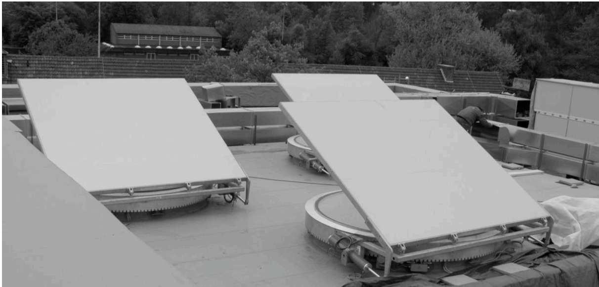
Figure 4: Rooflight heliostats at the construction site of the Science College Overbach
