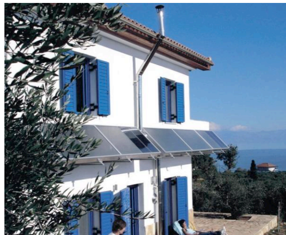
Figure 6: Renovation of a 2 nd home in Koroni GR with a pv-powered solar air collector (Grammer Solar AG)
