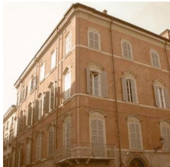
Figure 2: Historic villa in Modena IT renovated with interior insulation (V. Calderaro)
