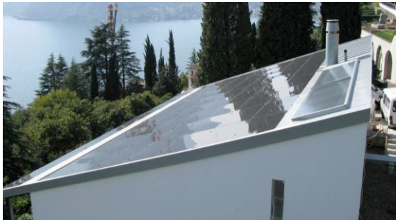
Figure 1: mono crystalline BiPV plant in Ruvigliana (TI-CH, photo courtesy of Ecosinergie).
