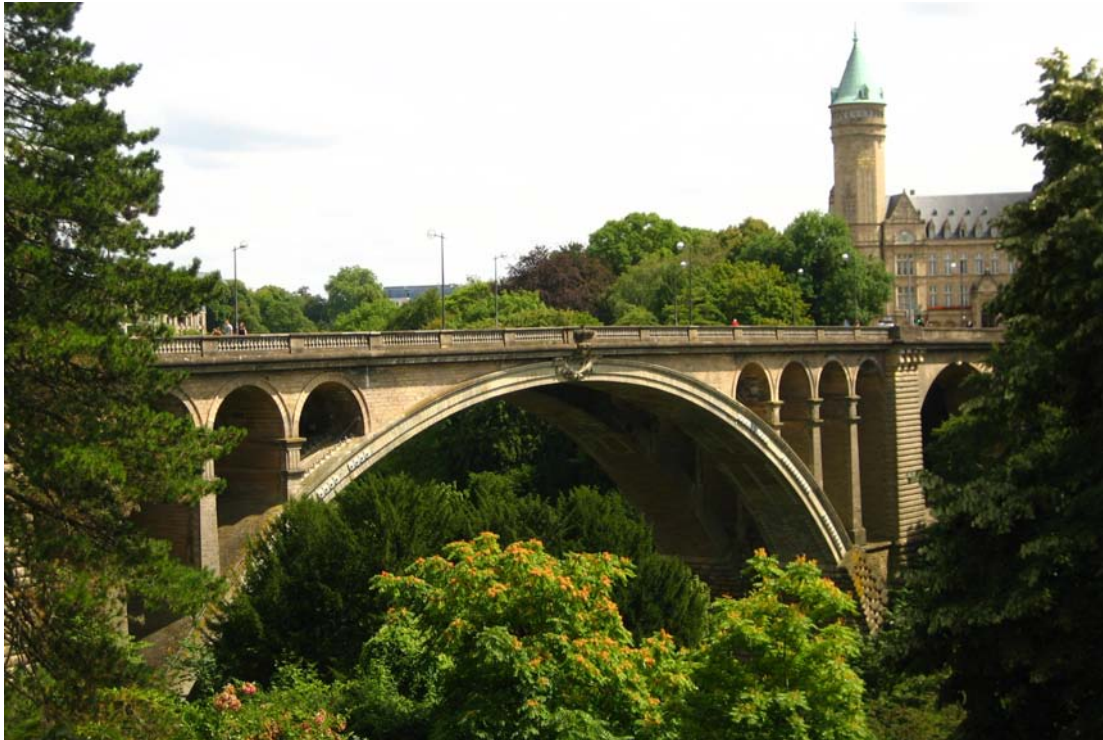
Figure 2.14 : Pont Adolphe, Luxembourg
