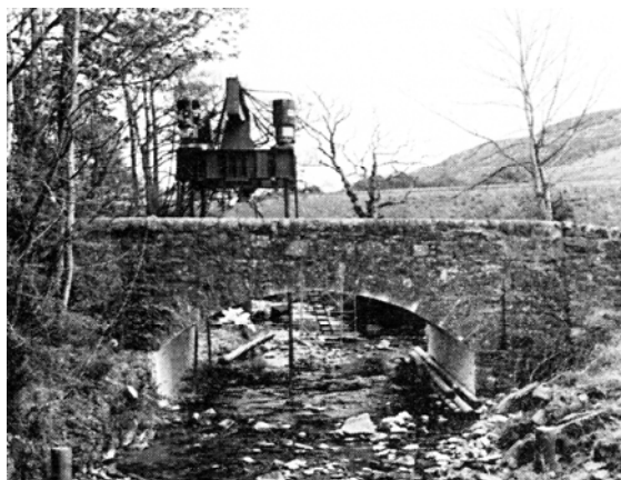
Figure 7.16 : Le Shinafoot Bridge [7.1]
