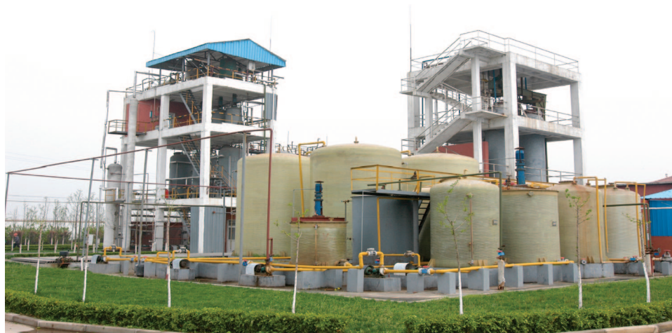
Figure 1. Demo-plant of ethanol production from lignocellulosic biomass.
