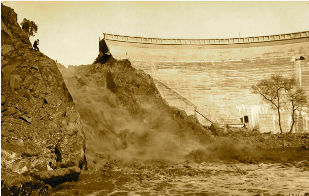
Figure 1.1: View of the break in Sweetwater Dam (Jan 30, 1916). ©San Diego Historical Society ( http://www.sandiegohistory.org )
