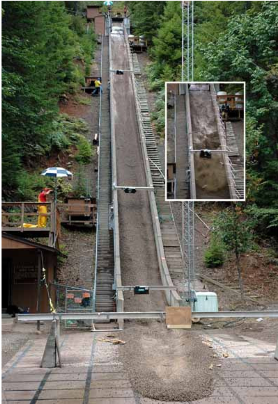
Figure 1.2: Flume constructed in 1991 by the U.S. Geological Survey (USGS), in cooperation with the U.S. Forest Service, to conduct controlled experiments on debris flows (Logan and Iverson, 2007): The flume is a reinforced concrete channel 95 meters long, 2 meters wide, and 1.2 meters deep that slopes 31 degrees (60 percent), an angle typical of terrain where natural debris flows originate.
