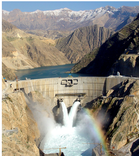
Figure 1.1: Francis hydropower plant Karun III, 2'000MW, South of Iran
