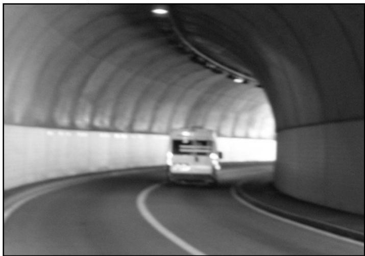
Figure 4-17: Jaun Pass tunnel - Looking west through tunnel.
