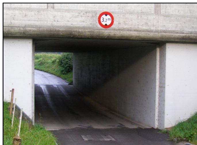
Figure 4-4: Eastern elevation of the exposed A2 bridge.
