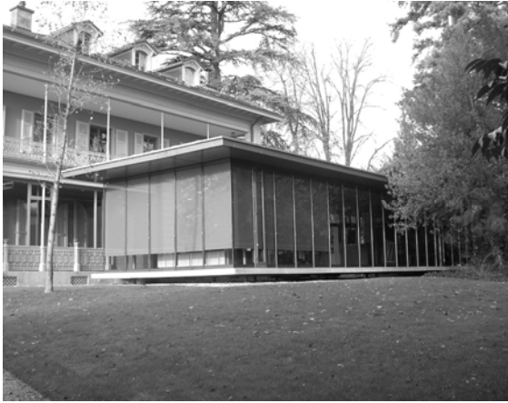
Figure 2.18 –Hermitage Museum, Lausanne (CH)
