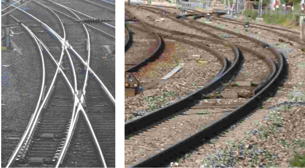
Figure 19 Left: Special curved diamond crossing with single slip in Bern (CH). Right: Curved standard left hand turnout in Palézieux (CH)
