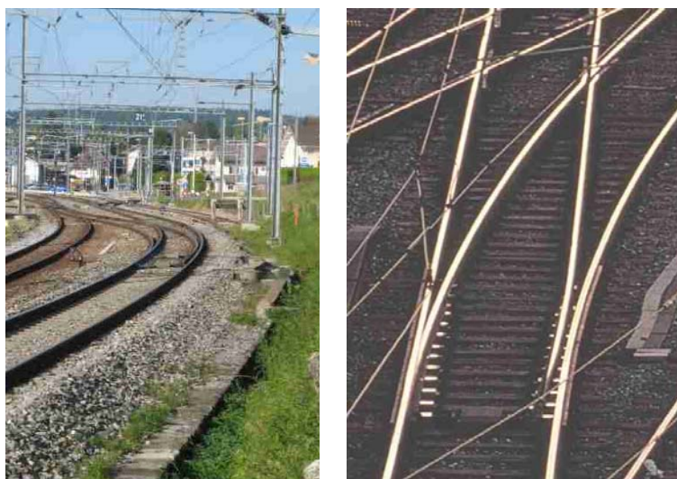
Figure 54 On the left a curved turnout (both directions are in a left turn), on the right a top view on a normal turnout with one straight direction and one curved direction
