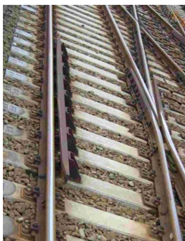
Figure 27 Check rail on the left, opposite of the frog on the right, Rotterdam (NL)
