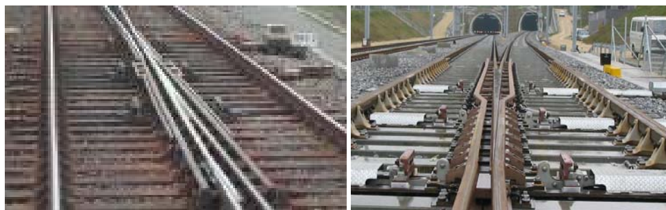
Figure 26 Left: Swing nose crossing, Amsterdam (NL) 19 and Wanzwil (CH) 20
