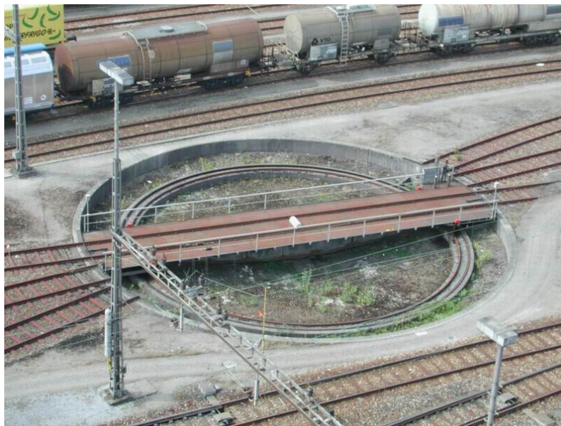
Figure 3 Example of a discontinuous way of changing tracks: a turntable in Muttens (CH)
