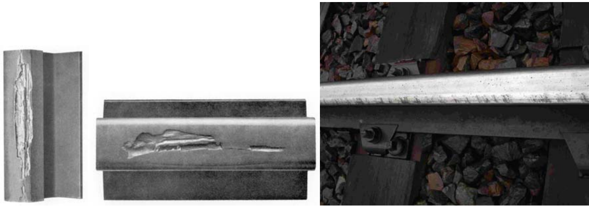
Figure 41 Examples of rail wear. From left to right: Gauge corner defect, running surface defect and head-checks (last one: junction of St. Benoit (F))
