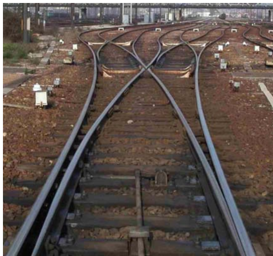
Figure 10 Symmetrical turnouts, marshalling yard of Villeneuve (F)
