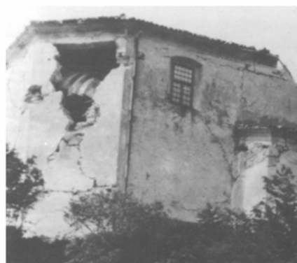
Figure 16.18 : Damage observed on the apse after both seismic tremors.
