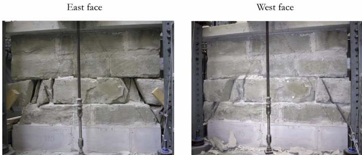
Figure 7.11 : Crack patterns on the east and west faces at the end of the 11‰ cycles.
