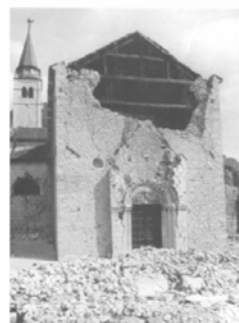
Figure 16.28 : Front wall damaged by the main seismic shock occurred in May 1976.
