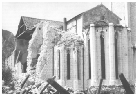
Figure 16.31 : East side of the dome after each seismic tremor.
