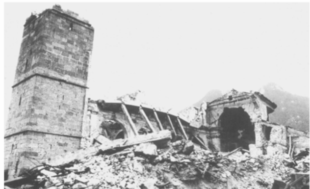
Figure 16.13 : Observed damage to the fabric of the church after the main (left) and second (right) seismic event.
