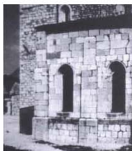
Figure 4.35 : Detachment of a part of masonry belonging to the outer leaf wall caused by the earthquake (Duomo di Venzone).
