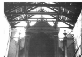
Figure 16.30 : Separation of the front wall belonging to the north transept.
