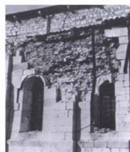
Figure 4.35 : Detachment of a part of masonry belonging to the outer leaf wall caused by the earthquake (Duomo di Venzone).
