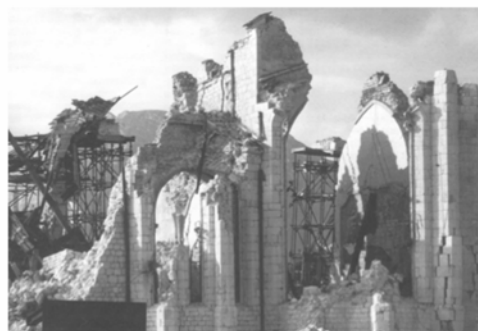
Figure 16.31 : East side of the dome after each seismic tremor.
