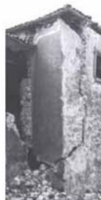
Figure 4.41 : Damage caused to a corner of a church due to the thrust from a roof rafter.
