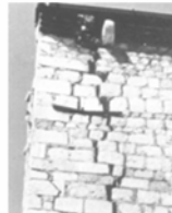
Figure 16.30 : Separation of the front wall belonging to the north transept.
