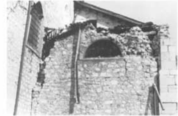
Figure 4.42 : Impact on the damage, following an earthquake, due to the adjunction of an appendix (Duomo di Venzone) [Do 94].
