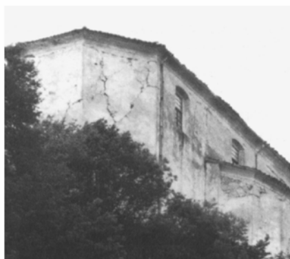
Figure 16.18 : Damage observed on the apse after both seismic tremors.
