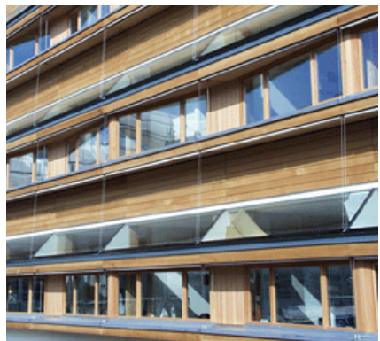
Fig 1.18 → An anidolic system integrated into the LESO solar experimental building on the EPFL campus (Lausanne, Switzerland) (1999)
