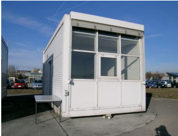
Fig. 3.1 External view of the real building (south facade)
