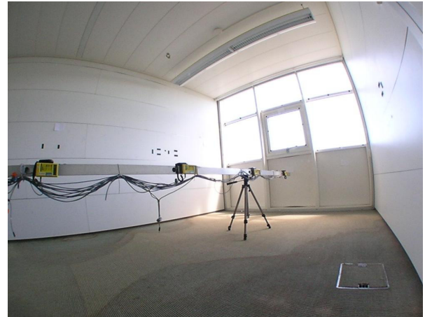
Fig. 3.2 Internal view of the real building towards the south facade
