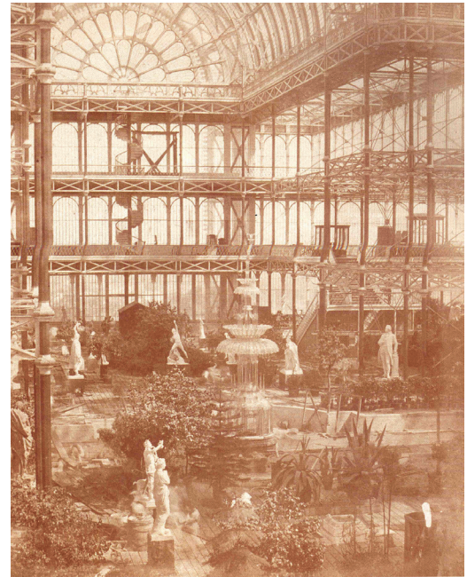
Fig. 1.7 Modular cast iron columns and beams allowed the composition of the transparent Crystal Palace, Great Britain, in industrial times (1851-1963)
