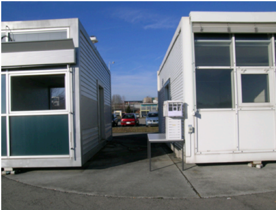
Fig. 5.30 Scale model location close to the real building (fixed to its western side)
