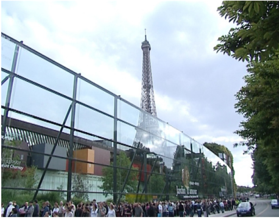
Fig 2.30 Glass fenestration of the Branly museum, Paris, France
