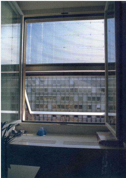
Fig 1.17 Prismatic panels on the CNA-SUVA building, Basle (1993)
