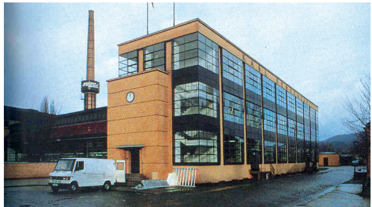
Fig. 1.8 Glass curtain walls of the Fagus Factory, Germany (1909)
