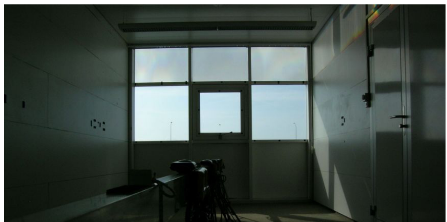
Fig. 3.26 Prismatic film fixed to the windows above eye level in the real building
