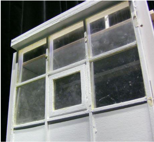
Fig 2.32 Dirt can reduce glazing transmittance
