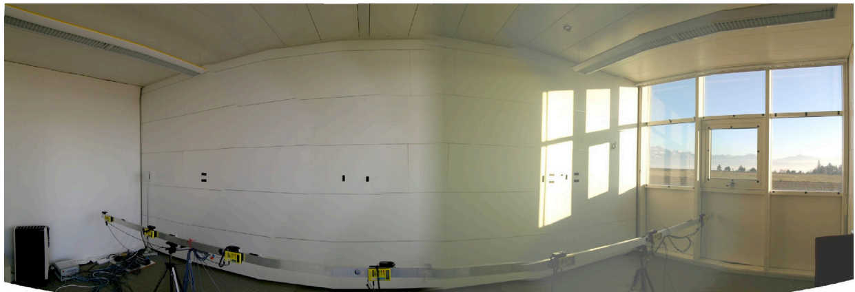
Fig. 3.14 Surface reflectance of the real building (photo)
