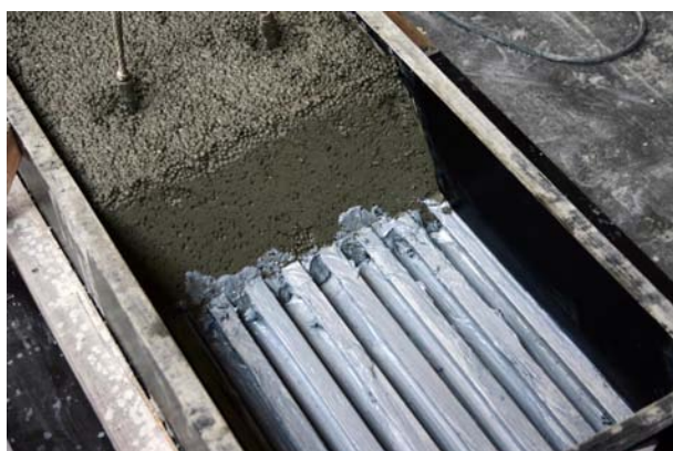
(a) Epoxy adhesive on GFRP profile
