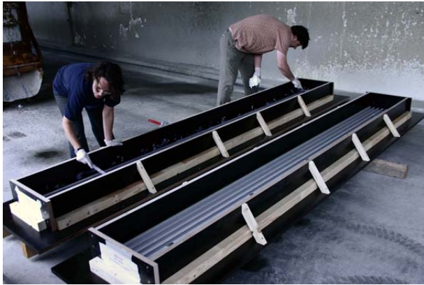
(a) Applying epoxy adhesive
