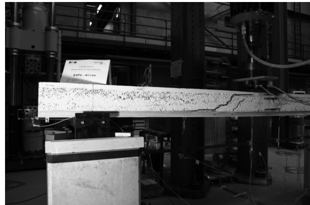
(d) Cracks at ultimate load at 42.8 kN and 12.3 mm deflection
