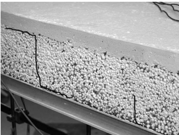
(e) Debonding at 8.4 kN (post-peak) on north west side
