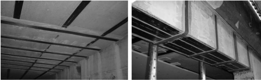
**Figure 2.2:** Duttweiler Bridge, Switzerland. Left: strengthening of deck slab with crossed CFRP strips, anchoring of transverse strips in cross-beam. Right: strengthening of cross-beam with strips and crossed L-shaped plates, taken from [Kel03].
