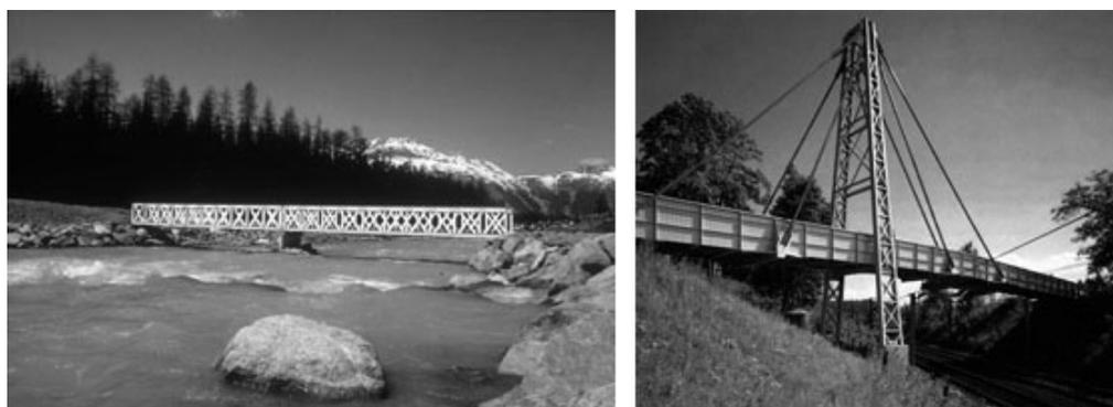
**Figure 2.4:** All-composite footbridges. Left: Pontresina footbridge in Switzerland, 1997. Right: Kolding footbridge in Denmark, 1997, both taken from [Kel03].
