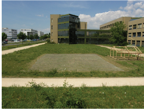
Figure 3-8 Ground plane installation at EPFL
