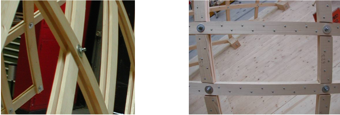
Fig 4 Intersection points before (left) and after (right) assembly of the intermediate in-fill layers
