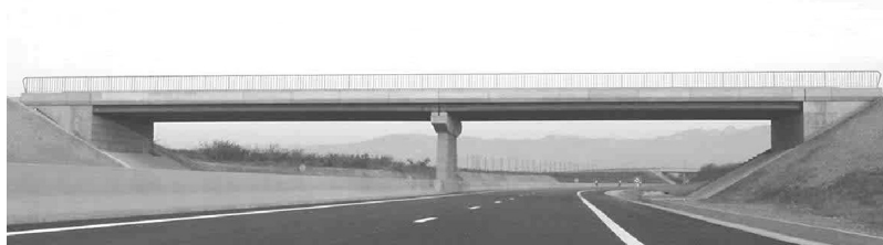
Figure 7.3: Bourg-lès-Valence road bridge: a) view on the two-span structure ; b) repetitive element of cross section ( \pi -shaped prestressed beam [Thibaux, Tanner 2002])
