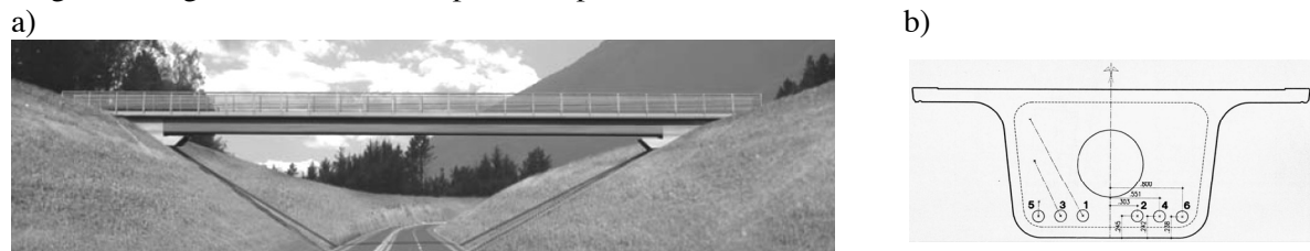
Figure 7.6: Bridge at La Chabotte, France, France: a) view of structure; b) cross section of bridge, [Resplendino, Bouteille 2006]
