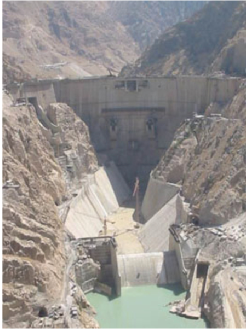
Figure 1.1.: Karun III arch dam in Iran, H = 205 m, maximum discharge capacity of 18'000 \text{ m}^3/\text{s} through chute and overfall spillways and orifices. Photo courtesy of Soleyman Emami of Mahab Ghodss Cons. Eng. Co., Tehran, Iran.
