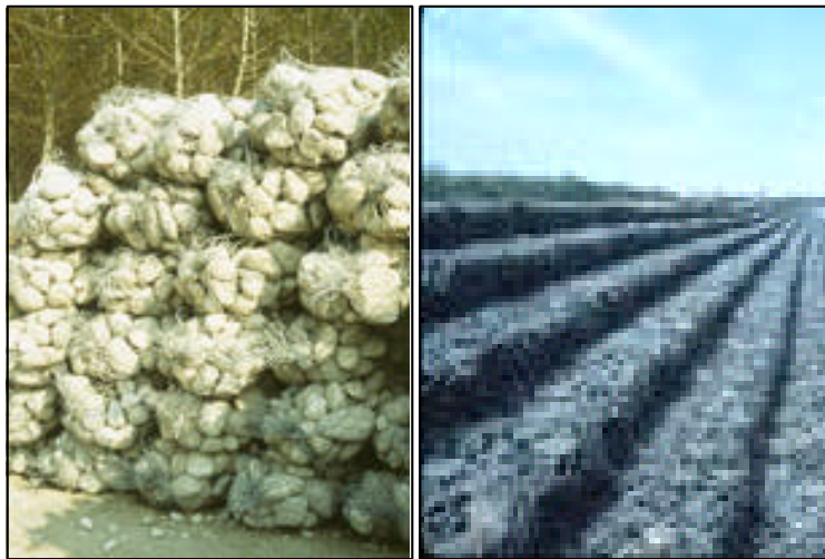
Figure 6.5: Left: Steel wire mesh baskets filled with stones; Right: Stepped Gabions protection - [Maccaferri (2004)]
