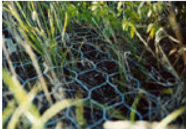
Figure 6.1: Establishment of vegetation within mattresses - [Maccaferri (2004)]
