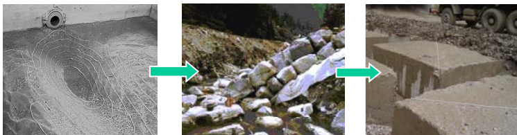
Figure 7: Alluvial bed (left), riprap protection (middle), concrete prisms (right)
