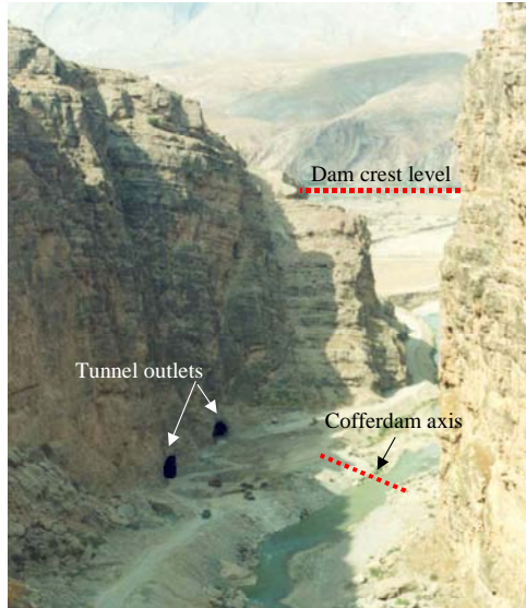
Figure 4: Downstream view of tunnel outlets of Seymareh diversion system
