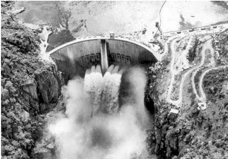
Photo 7 View from downstream to upstream of the Cabora-Bassa dam while discharging through 6 of the eight sluice gates.
