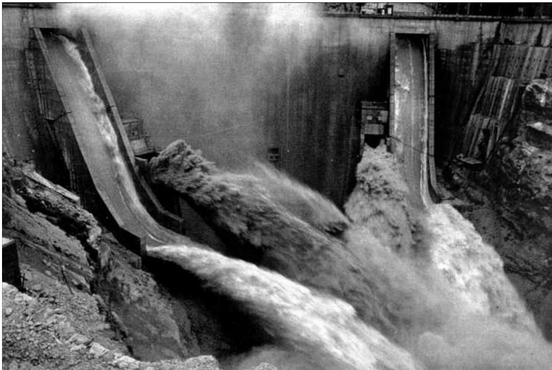
Photo 1 A 5'000 m 3 /s flood discharge at Jiroft dam (Iran): combination of highly sediment-laden flow, issuing from intermediate outlet works, with clear water coming from the ski-jump overflow structure (Photo B. Hagin, Stucky Ing. Conseils).
